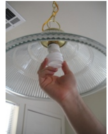
A CFL light bulb gets installed
